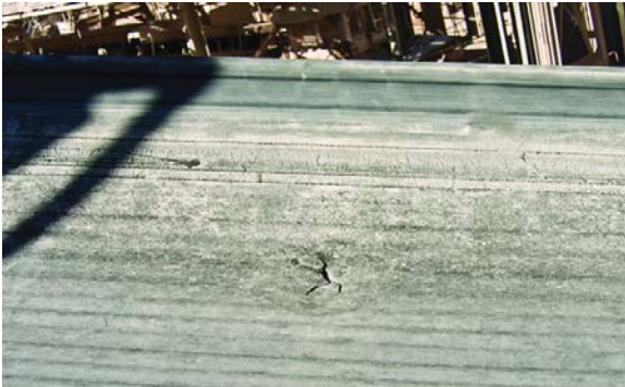
A receiving belt can experience severe damage from material transfers if it's not supported properly.
