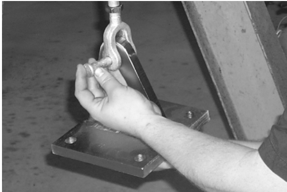
11. Assemble top mount weldment to turnbuckle.
