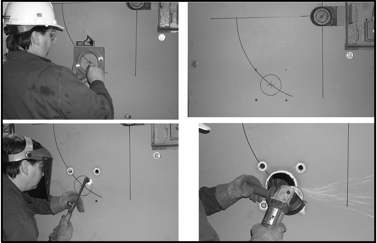
Figure 1. Belt Cleaner Mainframe Location & Chute Wall Cutouts
