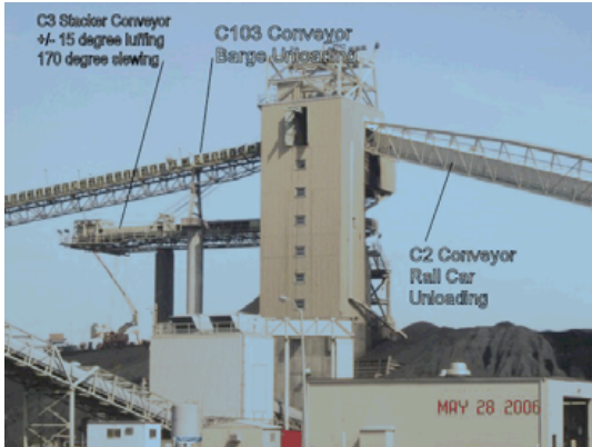
Two belts discharge at this transfer tower to feed the Rush Island C3 Stacker Conveyor.
