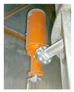
Martin® Air Cannons were installed on the silo to prevent the buildup of sugar on vessel walls.
