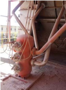
The Martin® Multi Valve Air Cannon improves flow at five discharge points.
