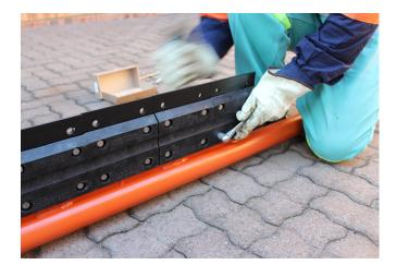
STEP 7: Continue working toward the centre by levelling two blades at a time. Tighten the bolts and nuts as you progress. Once completed and all the bolts and nuts have been tightened, test again with the straight edge to ensure that all blades are level.
