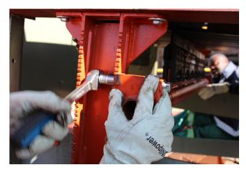
STEP 17: The lock nut on the adjusting bolt must now be fastened. All the bolts and nuts on the half clamps must now be fastened.
