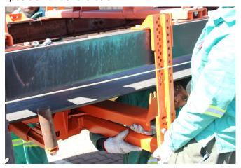
STEP 14: Install the idlers into the frames.
