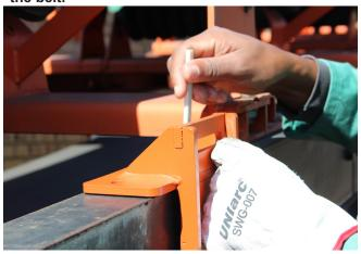
STEP 6: Secure the brackets to the stringer and tighten the bolts.
