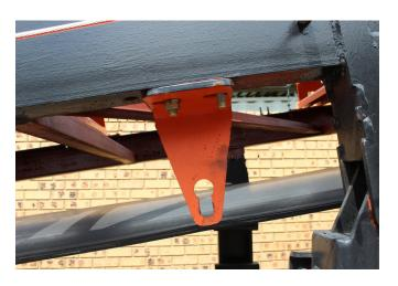
If neccesary mark new holes to be punched and punch or drill new holes.
