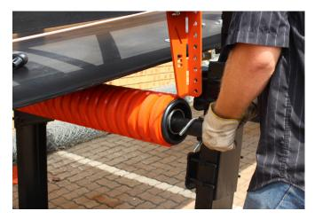
**STEP 7:**Place U bolt into holes on either side.
