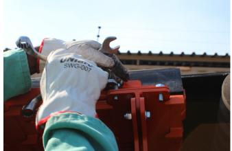
STEP 13: To ensure that the belt does not ride on the impact bars an idler frame must be placed before and after the impact bed to achieve this clearance. If the impact area requires that two impact beds be used, then an intermediary idler must be placed between the two beds.
