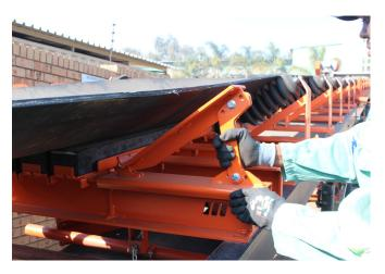
STEP 10: Slide the outer bars into position.
