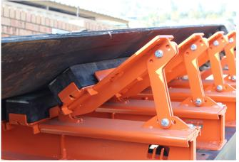
STEP 11: Insert the bolts and nuts into the wing support and tighten.
