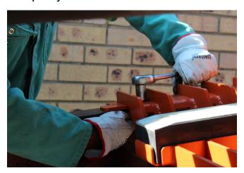
STEP 4: The lower weldment must be perpendicular to the structures and belt path. It must be centred in the middle of the structures.
