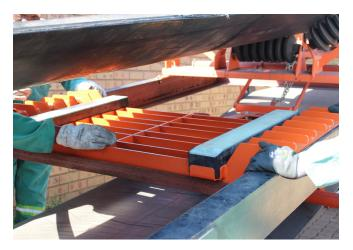
STEP 5: Mark all the fixing centres of the weldment. The structures must be cleaned of ant debris to ensure proper fixing of the unit.
