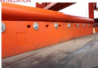
STEP 3: Drill or punch the holes as required. Secure the selected bracket to the structure
