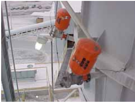
Martin® XHV Air Cannons are installed on the kiln at Mississippi Lime Company.
