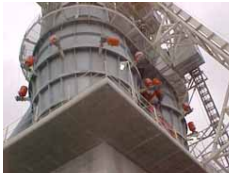
A total of 20 Martin® XHV Air Cannons from Martin Engineering were installed on the Maerz Kiln at Mississippi Lime Company's Ste. Genevieve Plant.
