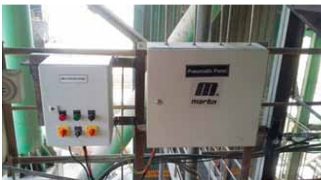
A solenoid box located far from heat & danger areas provides easy access.
