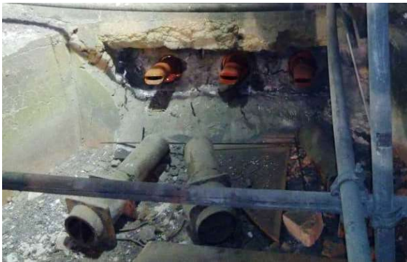
The old nozzles below had to be cut out, while the new orange ones simply slide out from the Y assembly.
