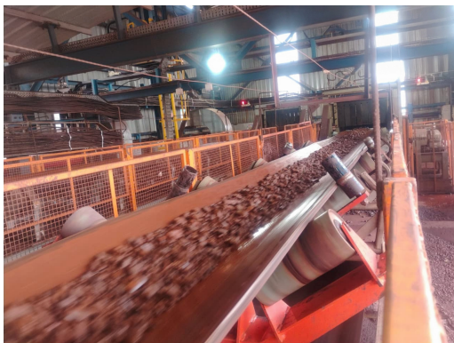
Belt sway was effectively eliminated, leading to a significant reduction in material spillage.
