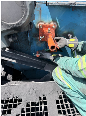
Installation of Martin® QC1+™ Cleaner HD
