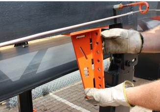
3. Ensure brackets is facing the correct way (arrow to point in the direction of the return belt).
