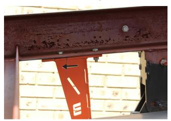
4. After holes have been punched, fasten brackets using M12 bolts & nuts provided.
