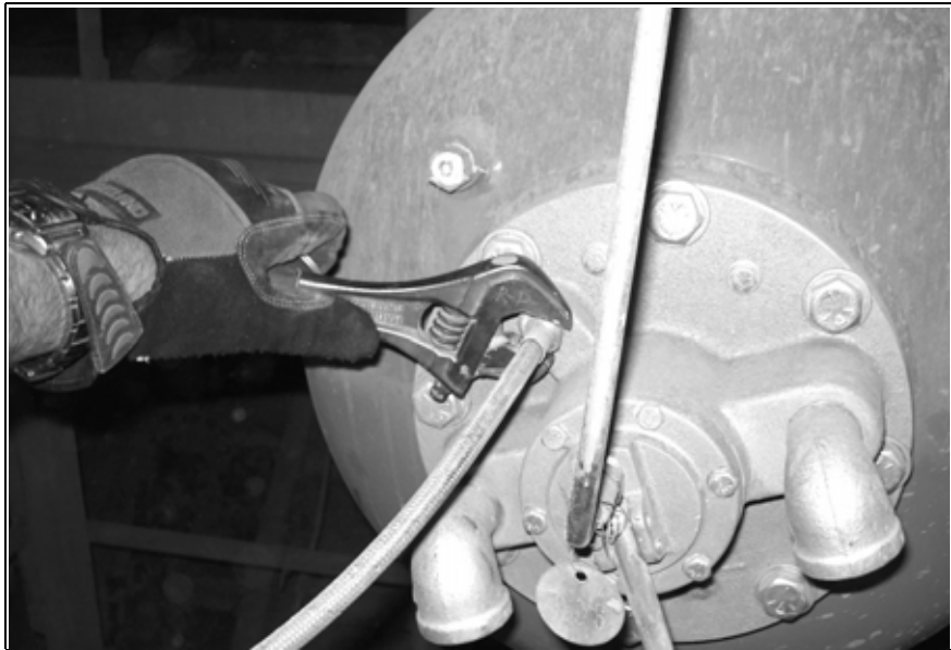
Fig. 22: Connecting the compressed air feed line
