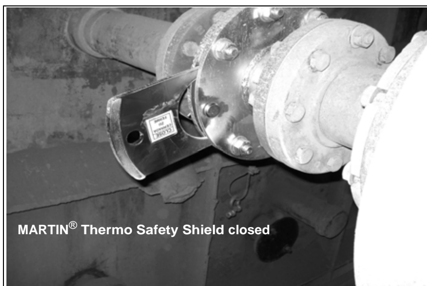
Fig. 13: Closing the thermo safety shield
