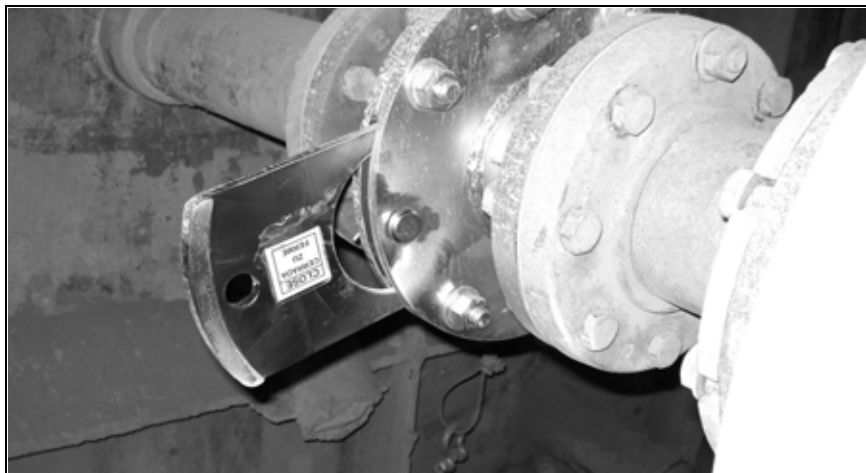
Fig. 23: Opening the thermo safety shield
