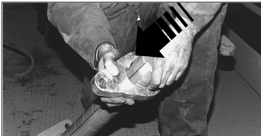
Fig. 2: Installing the shaft end stop
