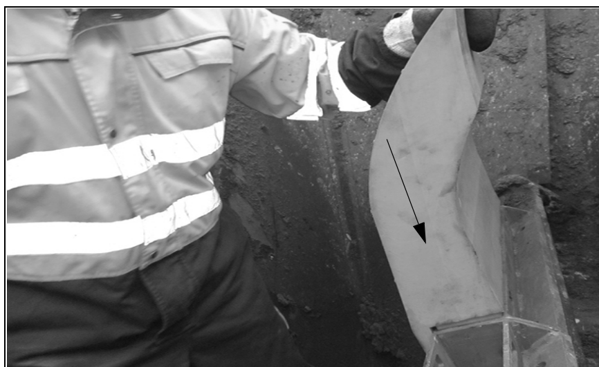
Fig. 11: Inserting the cleaner blade
