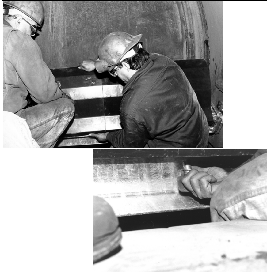
Fig. 8: Installation of the cleaner blades (1)
