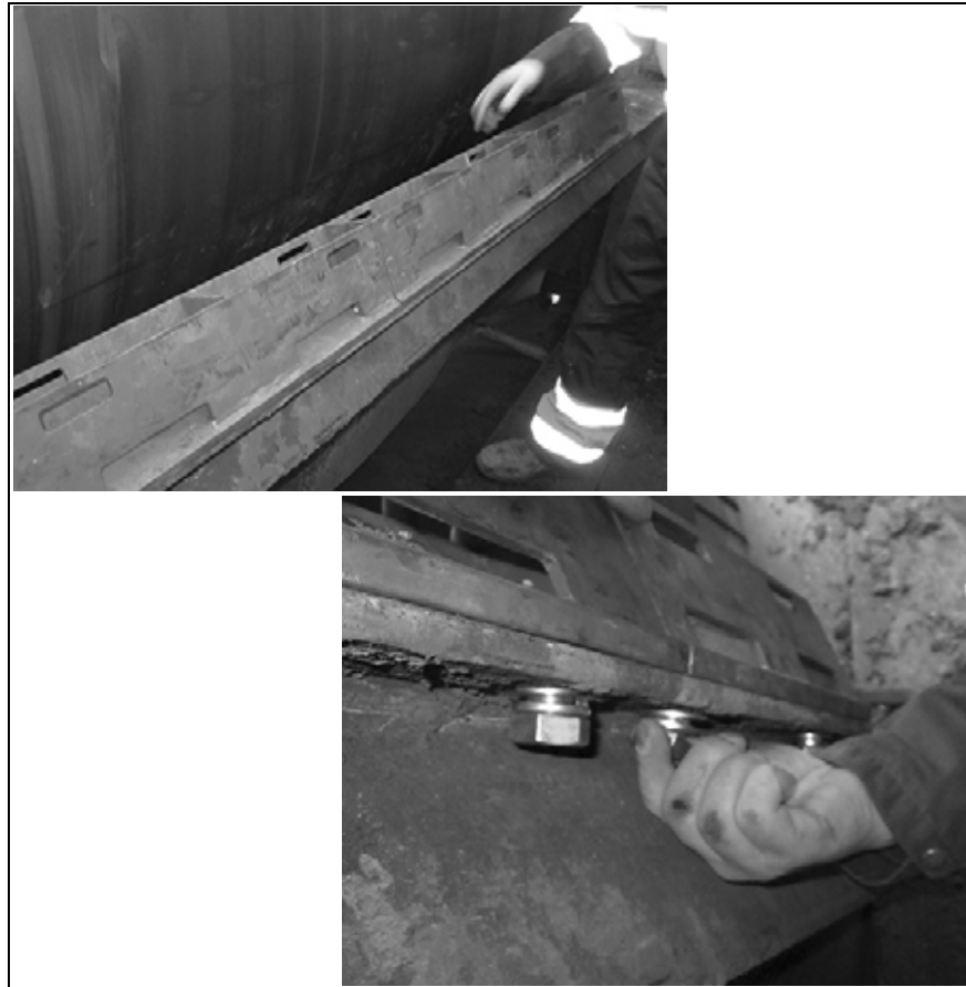
Fig. 10: Installation of the blade grip
