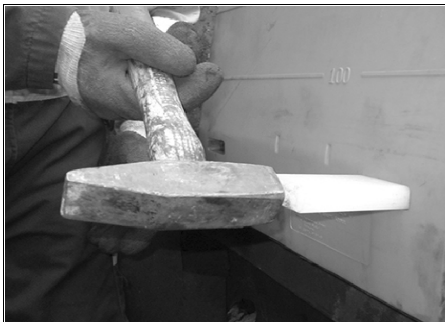
Fig. 12: Fixing the plastic pin
