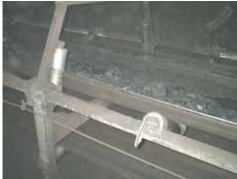
The conveyor system in SNSG's underground mines is suspended from the ceiling.
