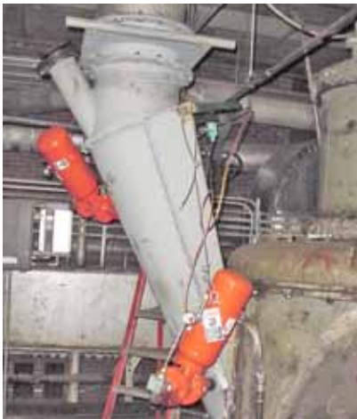
Air cannons are installed on the new chutes at Hennepin Power Station to prevent blockages.
