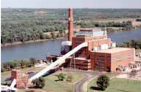
Hennepin Power Station
