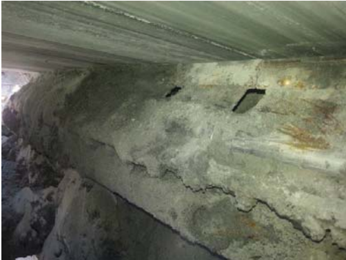
At a cement plant in Colombia, limestone was accumulating on the return roller and the underside of the belt.
