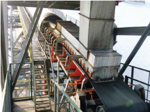
After assessing the design, Martin Engineering determined several areas for improvements.
