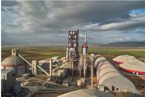
A cement plant in Turkey with the highest clinker production capacity was having problems with material flow.
