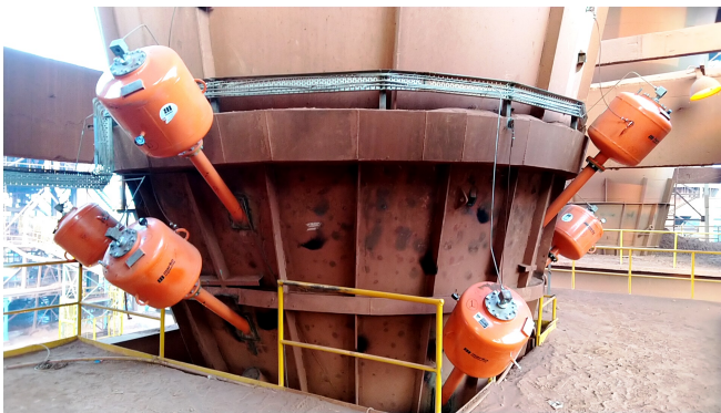
Strategically positioned at critical points around each silo, the Typhoon Air Cannons prevent accumulation.
