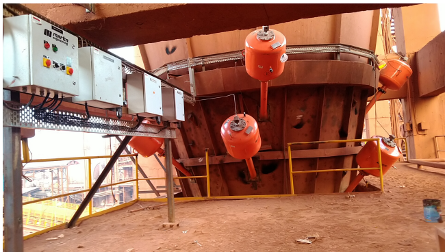
The air cannons can be programmed to fire automatically or manually activated as needed.
