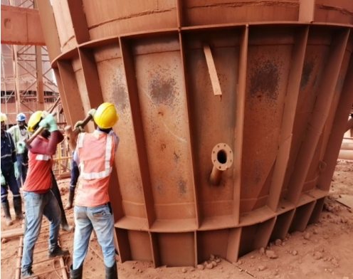
Maintenance personnel were manually hammering to dislodge blockages - causing damage to the silo walls.
