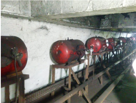
Continued coal buildup in bunker due to sticky material and ineffective blasters from another supplier
