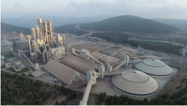
Medcem operates one of the world's largest and most important cement plants, exporting around 4 million tpa.
