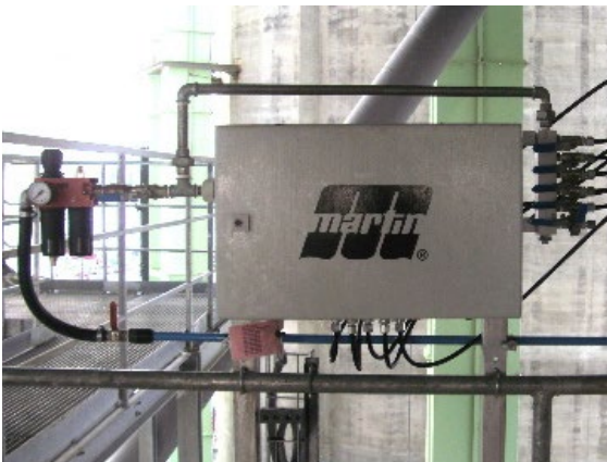
Solenoid valve cabinet installed in a protected environment
