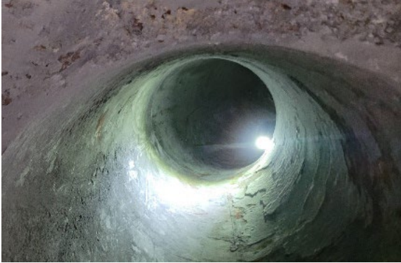
Flue gas duct cleaned with Martin® Hurricane air cannon
