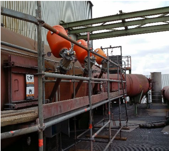
Air cannons on the flue gas duct
