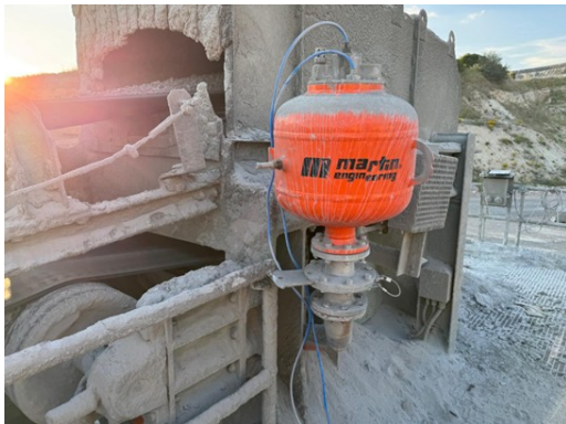
Following proven performance, the Air Cannon solution was replicated at additional transfer points.
