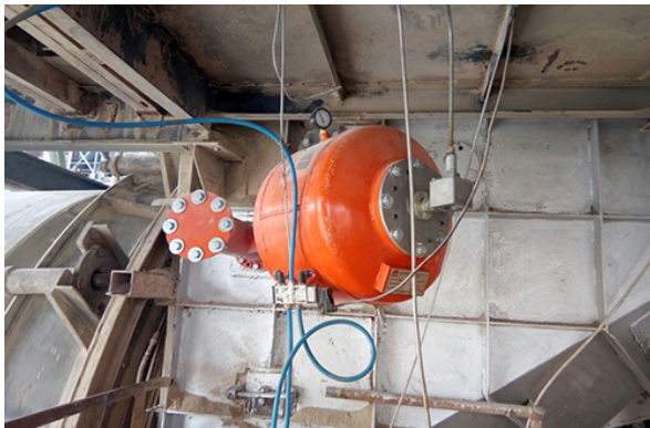
The outward facing valve and Y-pipe assembly is designed for ease of access and worker safety.
