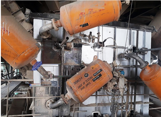
The large air cannons taxed the compressed air system, but accumulation remained a problem.
