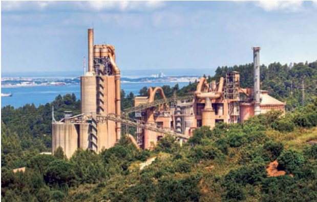
Secil Outão was experiencing severe build-up issues in the kiln inlet, smoke chamber, calciner, and cyclones.
