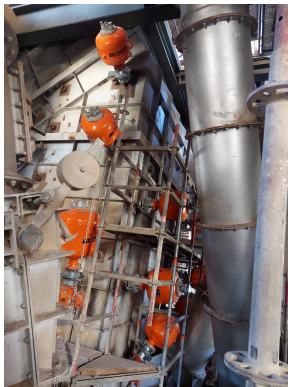
Total 67 Martin® Hurricane Air Cannons with varying capacities 35L, 70L, and 150L, were strategically installed
