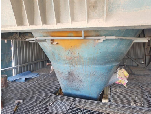
Fly ash hoppers faced frequent blockages. Vibrators and hammering proved to be unsafe and inefficient.
