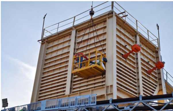
Martin® Hurricane Air Cannons Installation in progress
