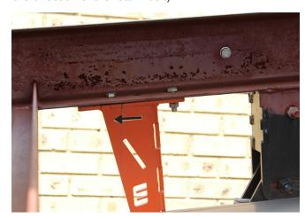
**STEP 5:** After holes have been punched, fasten brackets using M12 bolts & nuts provided.
