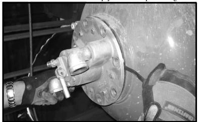
6. With the valve assembly removed, the rebuild can be done in the maintenance shop (see list of rebuild kits on page 30).
