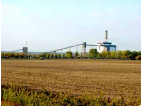
MidAmerican Energy Neal Station South
