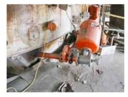
To reduce employee exposure to severe temperatures, Martin® Thermo Safety Shields were included in the air cannon installation project.
