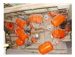
The elimination of the blockages required that the Martin® Air Cannons be "densely packed" on the pre-heater tower.
