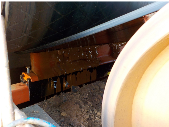
Operators report that blades run easily over the belt and splice and that the system is running efficiently.
