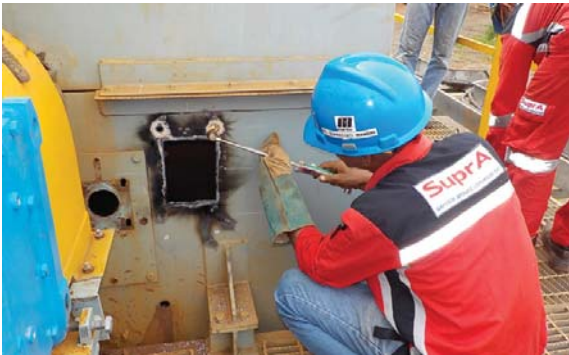
Technicians examined the issue and installed a Martin® QC1™ Cleaner HD and Martin® DT2 Inline Cleaner.
