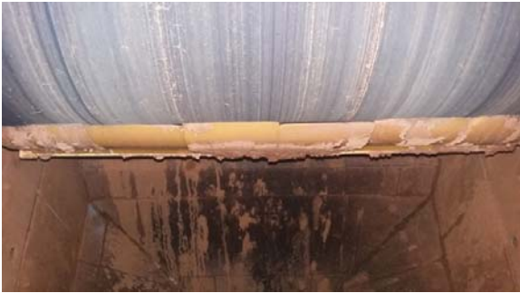
Rocks would wedge in the primary belt cleaner, breaking the splice and shredding the belt.
