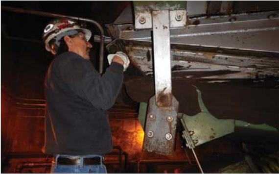
*Platte was experiencing failures of the rubber/fabric seals at the top of the chute wall on its train unload feeder.*
