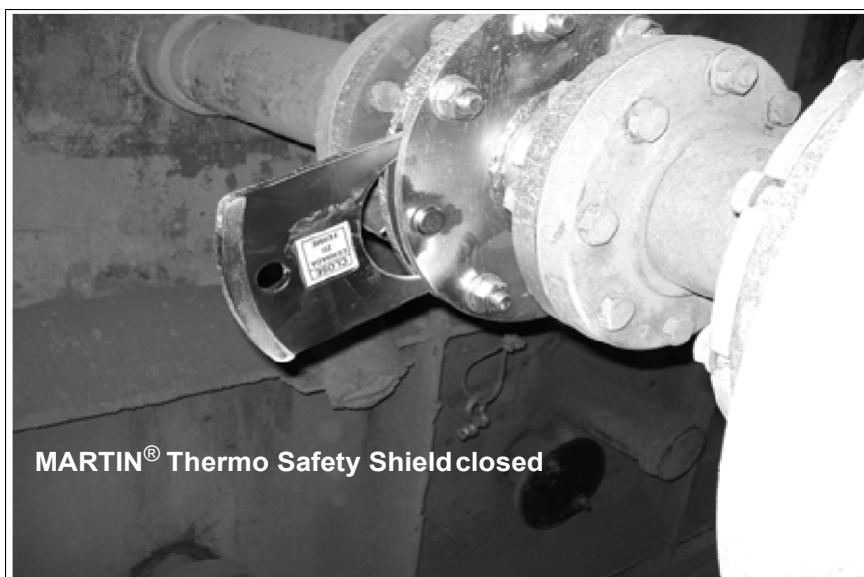
Fig. 13: Closing the thermo safety shield
