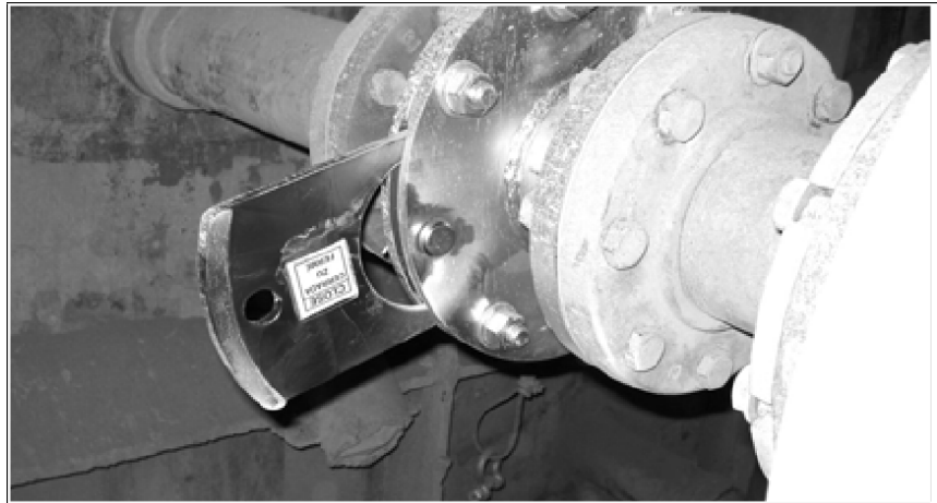
Fig. 23: Opening the thermo safety shield
