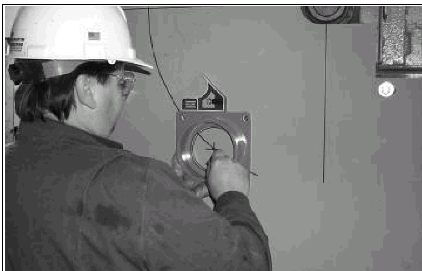
Abb. 4: Mark the axle opening and screw holes
