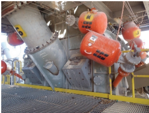
These cannons were positioned in the lower part of the pre-heat tower, near the automatic sampler.
