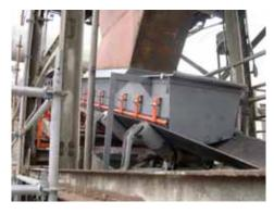
A Martin® Tail Sealing Box was fieldfabricated on each of the bark conveyors at Weyerhaeuser Pine Hill.
