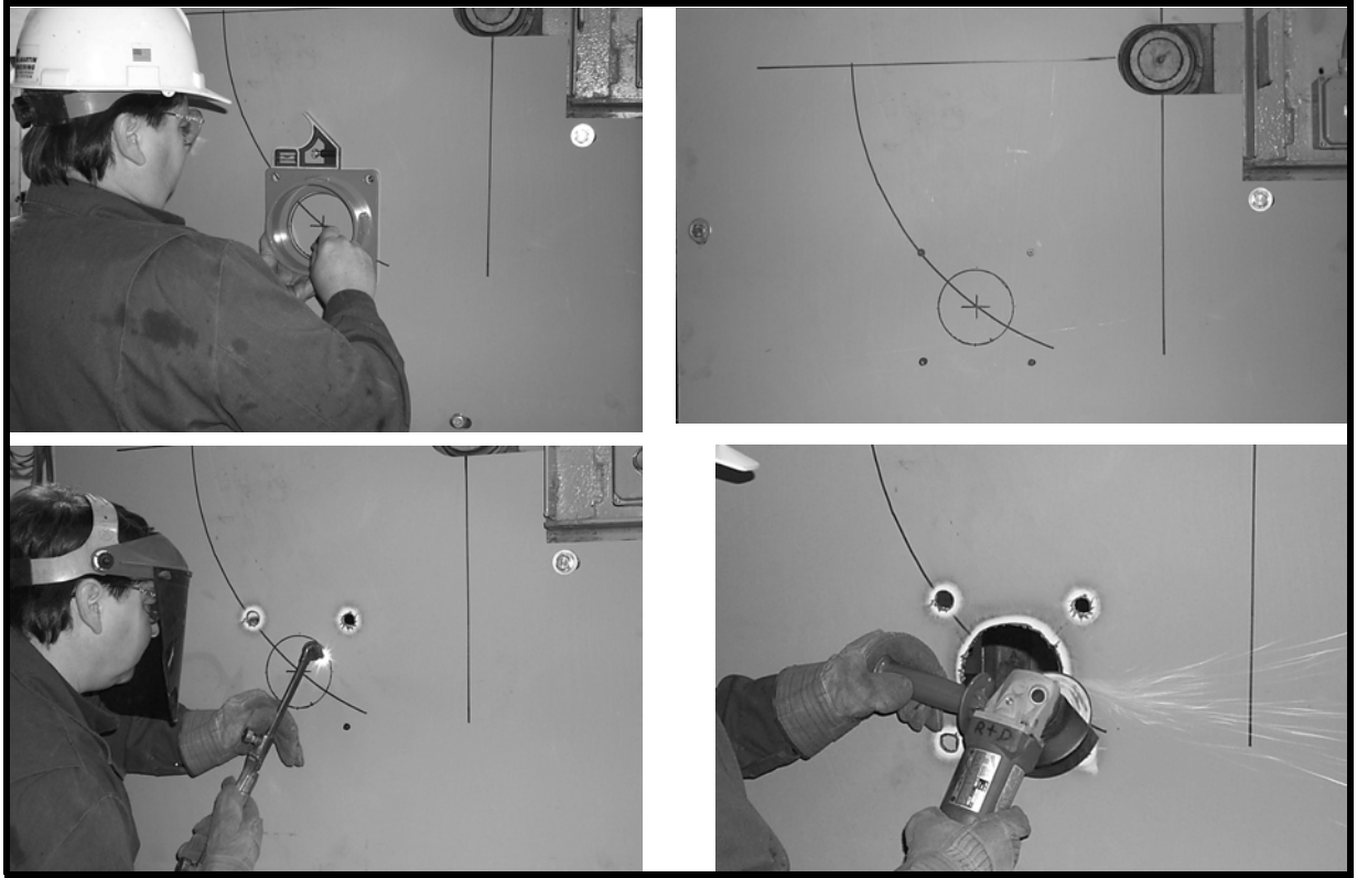
Figure 1. Belt Cleaner Mainframe Location & Chute Wall Cutouts
