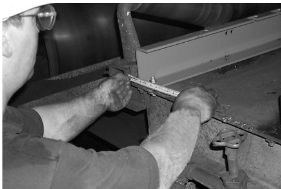
Figure 2. Installing Martin® Impact Cradles
