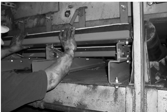
17. Install impact bars on wings.
