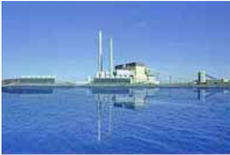
Alliant Energy power-generation facility, Lansing, Iowa
