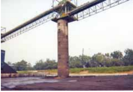
Six stacker tubes at the Kanawha River Terminals are used in the stockpile area to allow storage of coal.
