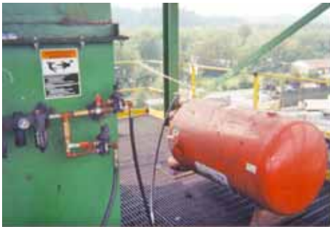
The Martin® Air Cannons were installed on the catwalk of the conveyors above the stacker tubes.
