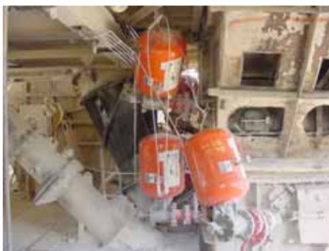
Martin® Air Cannons were installed on the pre-heater tower.
