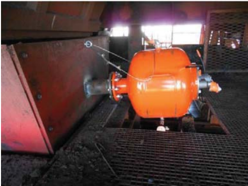
The solution was so successful, they are planning to add this solution to all of their transfer points in the facility.
